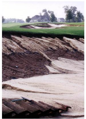
**Renovation** – Most closely synonymous with '*rejuvenate*', a bunker renovation can be classified as bringing conditions up to a desired level. This might involve minor drainage issues, liner installations, and sand replacement. In most cases, a bunker renovation is the least involved of the three.
